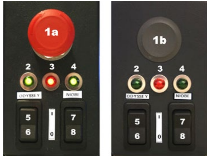
Figure 9. Vision Remote Power Box: Siemens labs (left), Philips labs (right)
